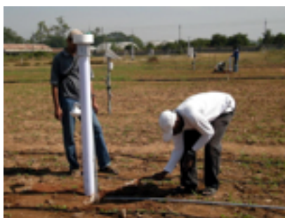
Field Server installation in Hyderabad, India
